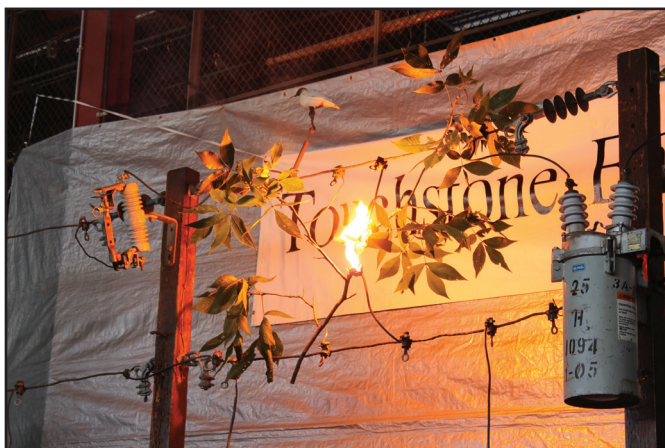
Live Line Demonstration
